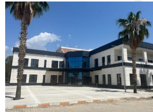
New R&D building
